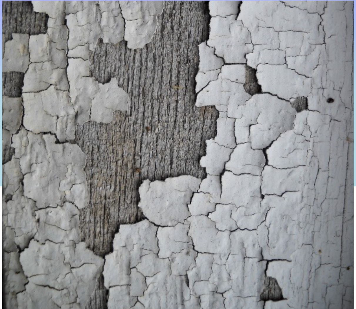
Image: chipping lead paint
